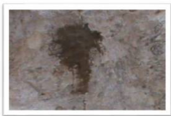
3. Covering the hole by moistened clay
